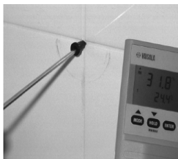
Fig. 1: Measuring humidity in a bathroom
